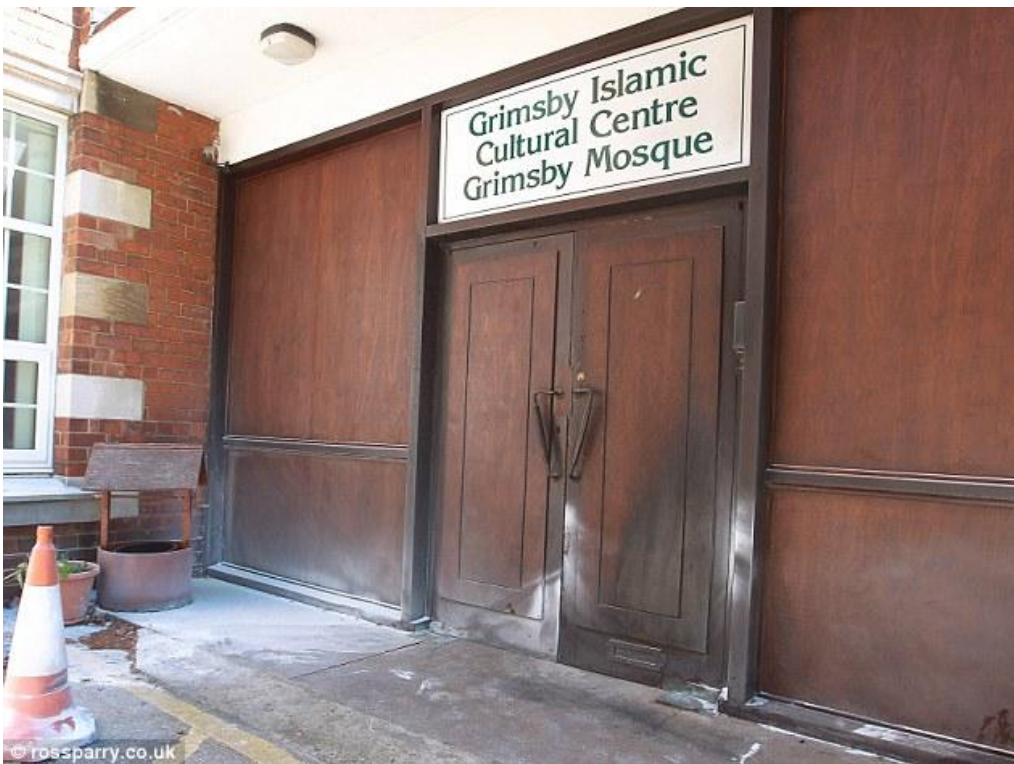
Attack: This scorched door to the Grimsby Mosque shows the damage caused by the firebomb attack last night
